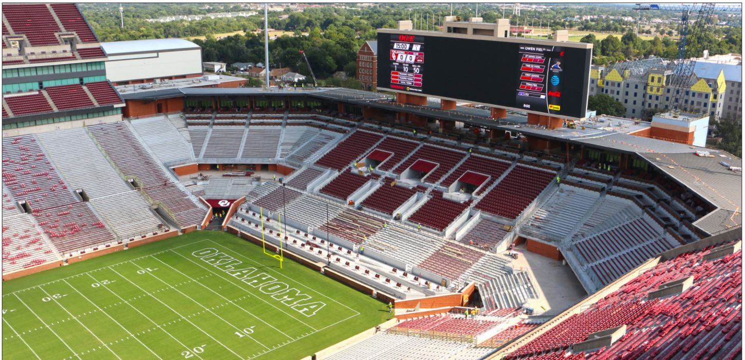
OU's $160 million stadium renovation and modernization project bowled in the south end of the facility and added premium seating and the second-largest collegiate video board.
